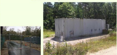
Demolition Area 1 Base Boundary and Off-base
